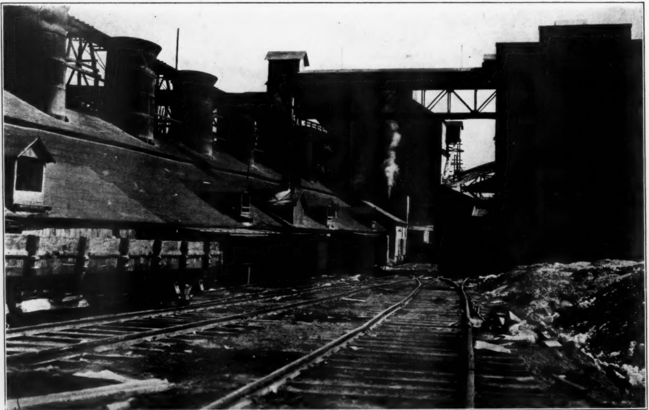
Kiln Battery on Left and Hydrate Building on Right. The Bridgework and Housing Shown in the Center is the Horizontal Conveying Unit for Transporting the Lump Lime to the Hydrator.
